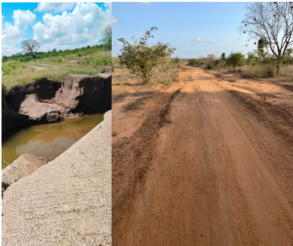
On the left one of the destroyed bridges, on the right the new road.
