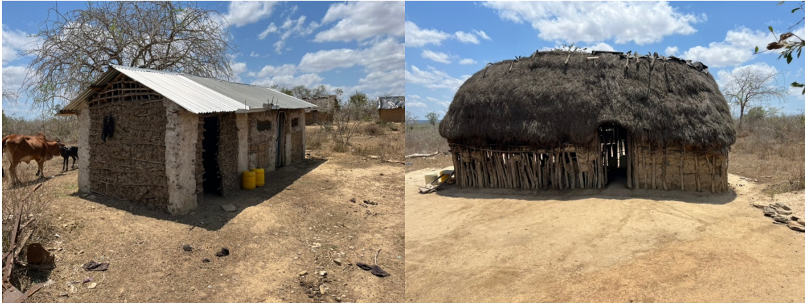
On the left the new goat shed, on the right the house of one of the members.
