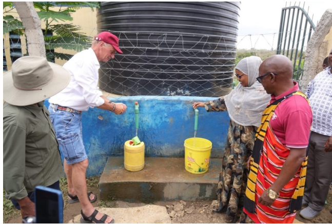
The opening at the water distribution point of Naserian.
